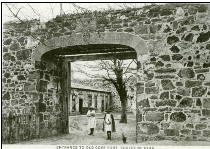
Keystone arch at Cove Creek Ranch Fort Erected 1867 (DUP Photo Collection)
