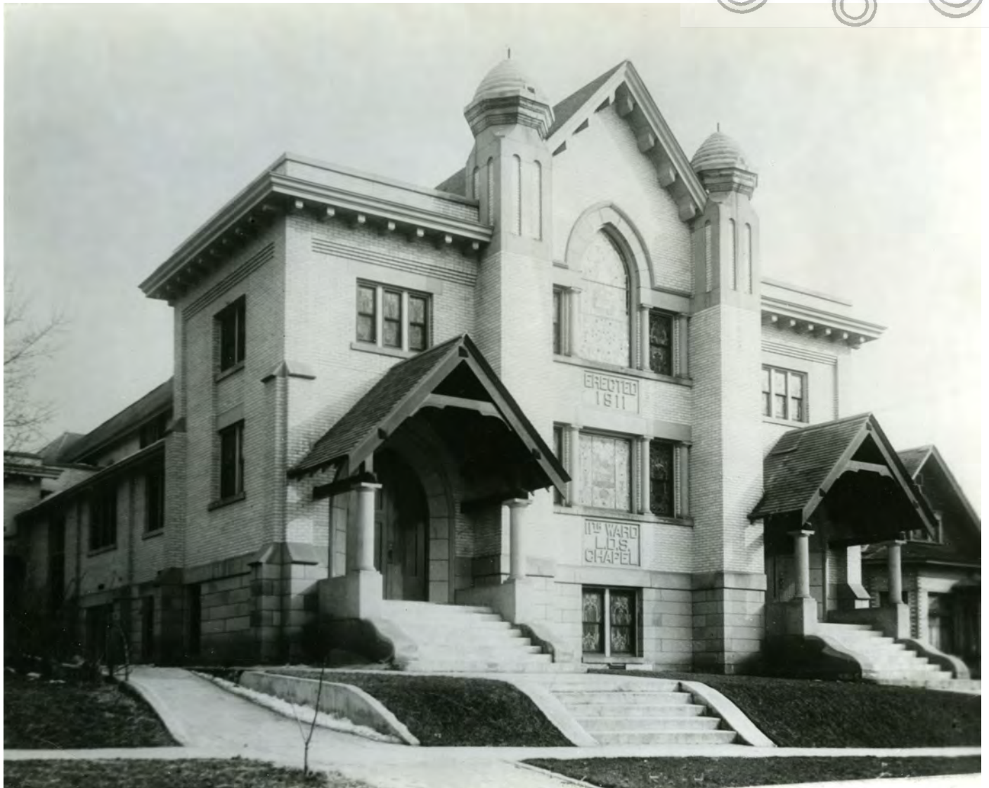
Eleventh Ward Building. (DUP Photo Collection)
