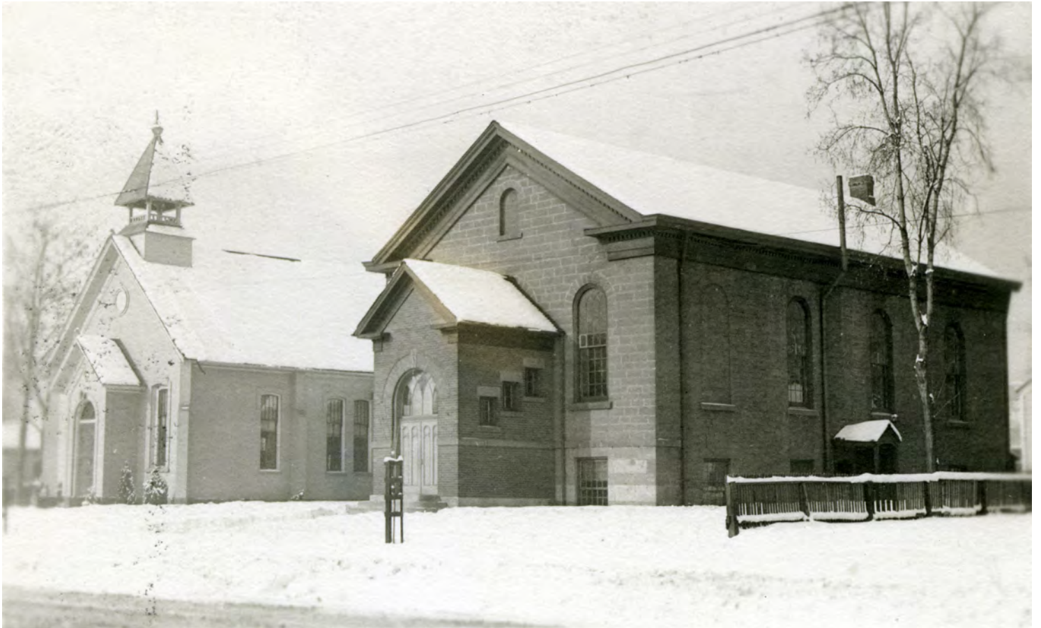
Seventh Ward building. (DUP Photo Collection)
