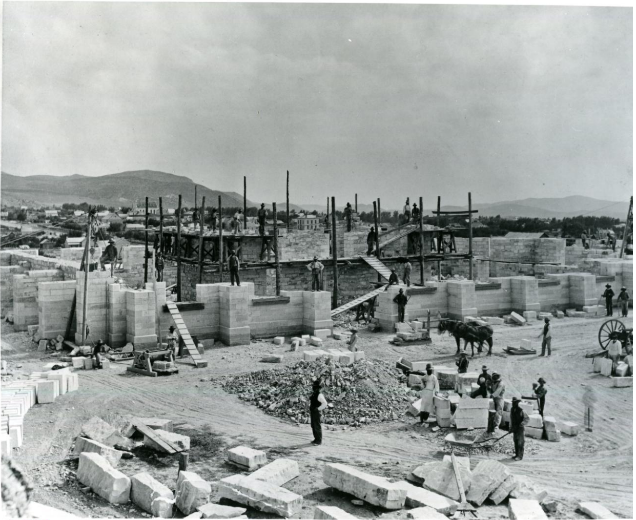
Salt Lake Temple construction (DUP Photo Collection)
