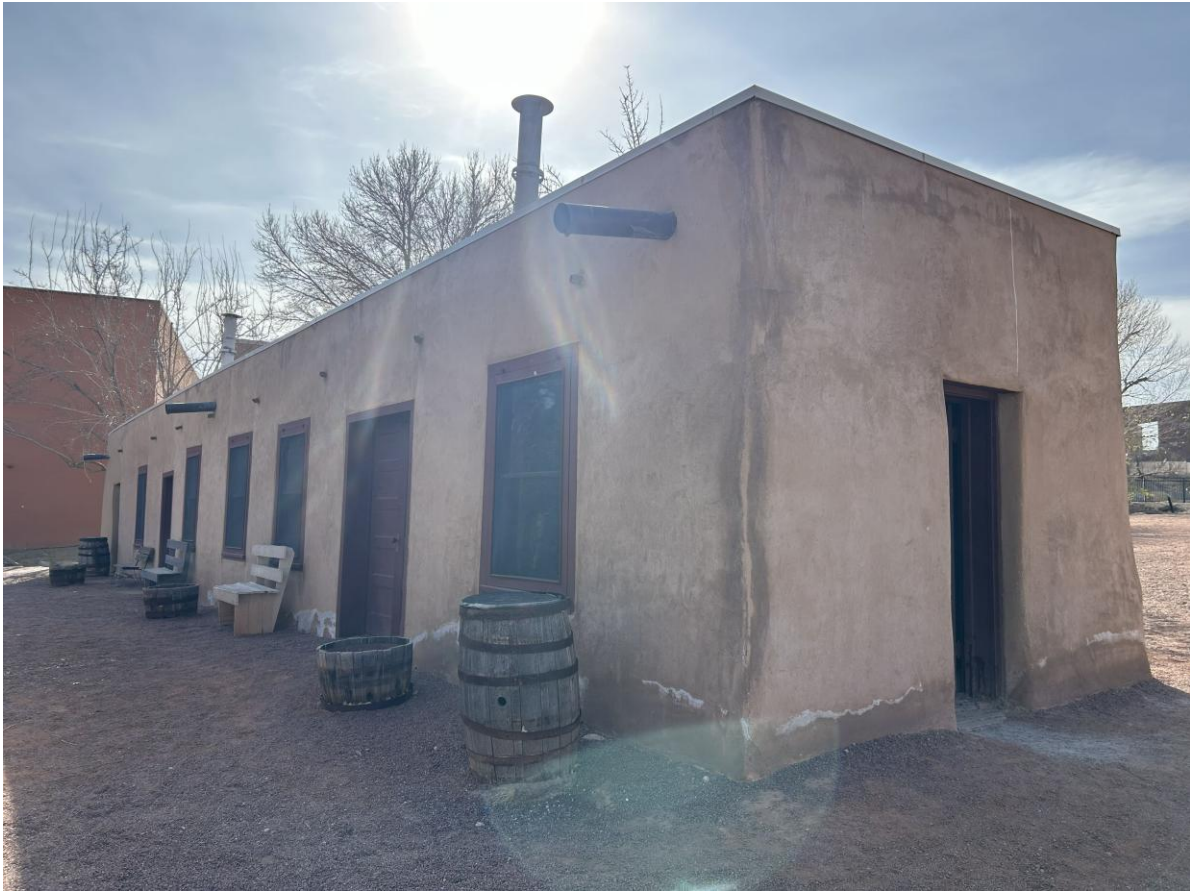
Nevada's oldest building. Old Mormon Fort State Park (Ellen Jeppson Photo)
